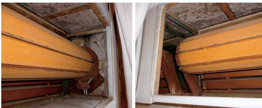
Figure 8 – Detail of the box and roll-down blinds
